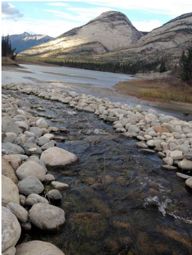
“Mile 9” TMLF project, Highway 16, near Jasper (credit: J.W. Bull)
